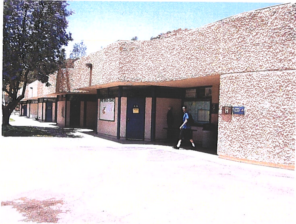
Classrooms - Buildings G and H
