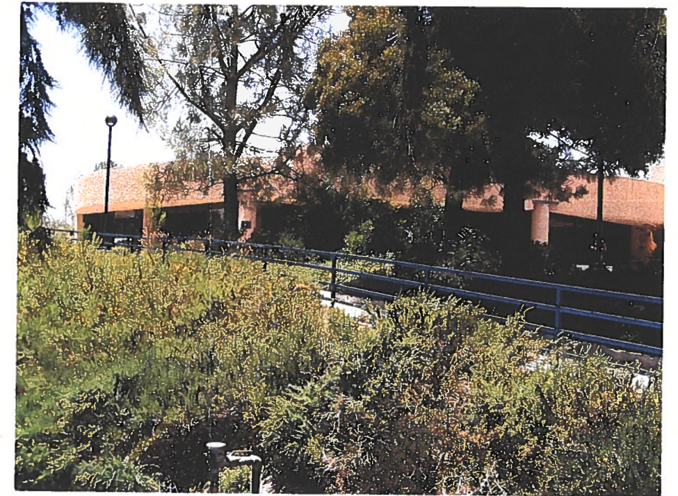
Classrooms, Administration and Student Services - Building N
